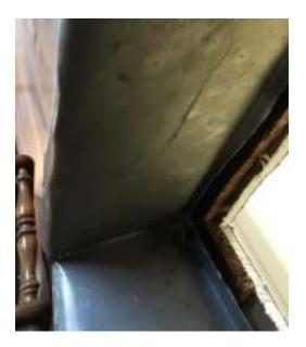
Ice dam problems have been noted on the older section of the building. A consultation with insulation professionals has been requested to advise on where the heat is entering the attic. Large gaps in the ceiling panel joints are visible. Tim screwed down the sheet metal and squirted in some foam insulation in the remaining gaps so at least we can address the bottom end of this issue.
